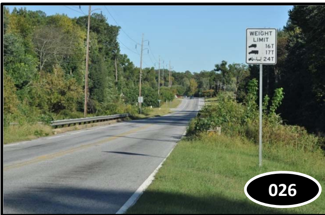
The bridge on Valley Hill Rd. at the Flint River in Clayton County will be replaced.
