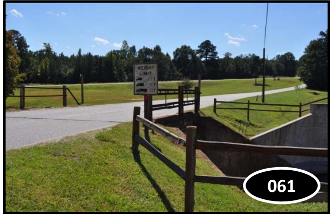
This bridge on Pylant St. and the nearby intersection with SR 16 in Senoia will be upgraded.
