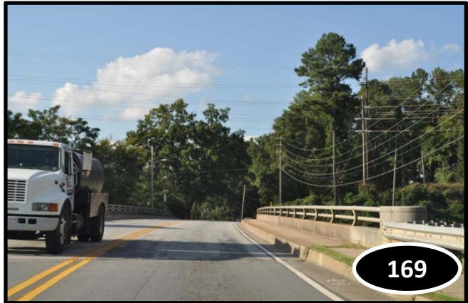
A new pedestrian bridge will be built, linking Oxford and Covington across I-20.
