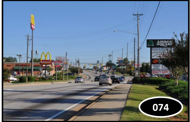
Safety and operational improvements will be made on SR 5 in Douglas County
