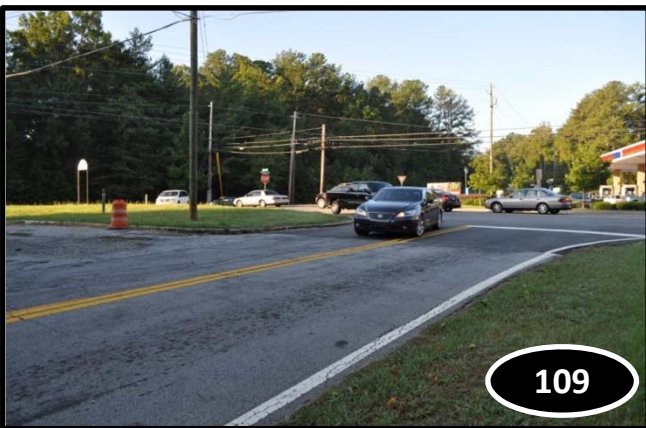
Sidewalks and a roundabout will be built at the intersection of SR 166 and New Hope Rd. in southern Fulton County.
