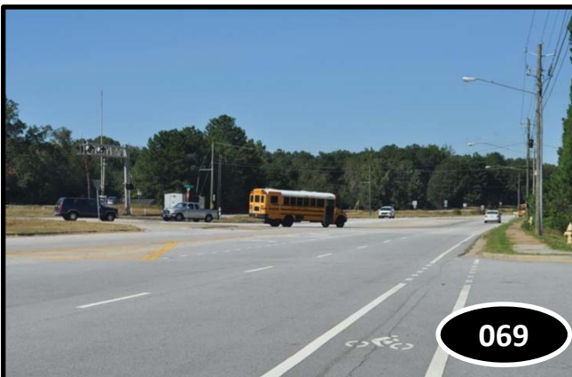
Scoping and engineering will be done to improve safety at the intersection of Panola Rd. and Stone Mountain Lithonia Rd. in DeKalb County.
