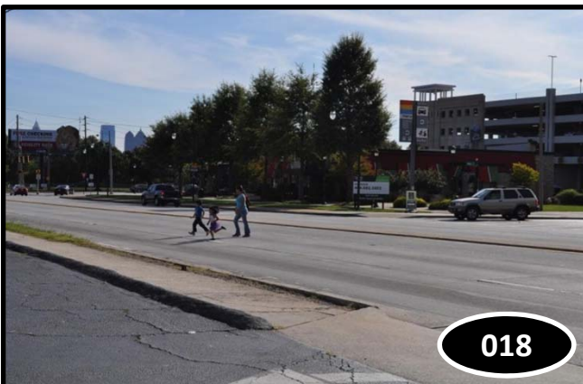
Pedestrian safety improvements will be scoped and engineered along Piedmont Rd. near the Lindbergh MARTA station in Atlanta.
