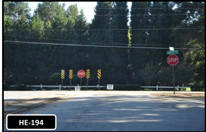
The intersection of Jodeco Rd. and Blackhall Rd. will be signalized.
