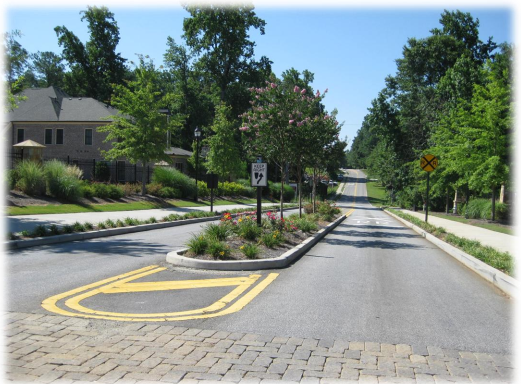
Street transition from a low volume, urban context to a rural environment
