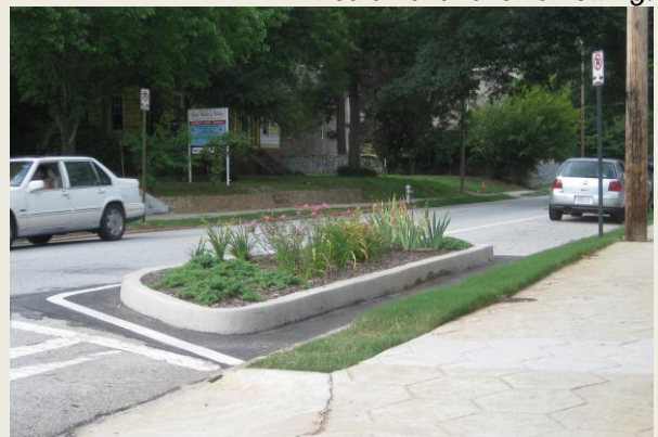
Curb extension slows down drivers.
