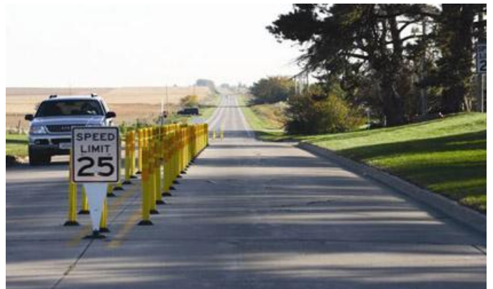
Median with tubular markers to help slow traffic. Photo credit: Federal Highway Administration.
