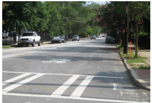
A narrow signals to driver that the roadway is intended for both bicycles and motorists.
