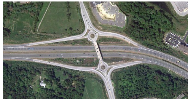
Figure 4.2 Double-roundabout interchange at Maryland Highways 100 and 103. Note that channelized right-turn bypasses of roundabouts are not pedestrian-friendly and increase the interchange's footprint.
