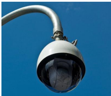
Figure 8-25: Traffic Operations Camera
