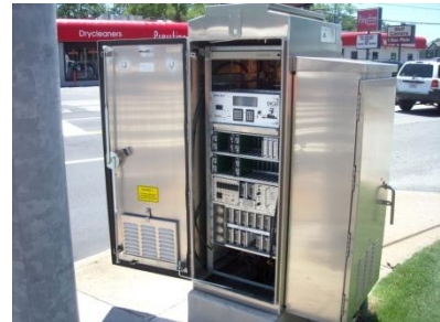
Figure 8-24: Signal Cabinet and Controller
