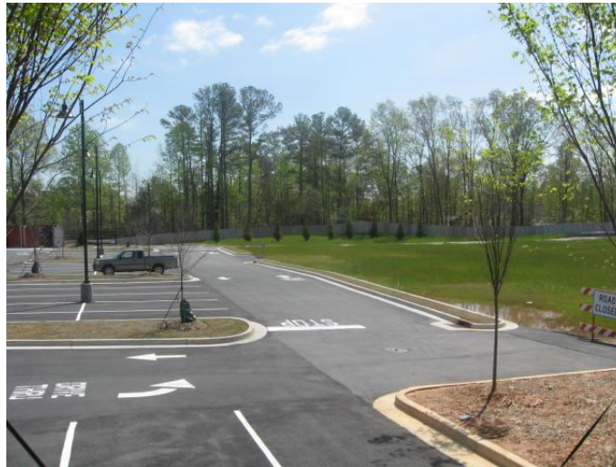
Figure 8-22: Stub Outs to Adjacent Land for Future Connections
