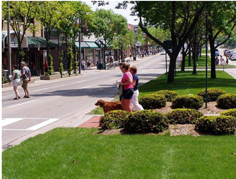
Figure 6-3: Raised Median with Pedestrian Refuge
