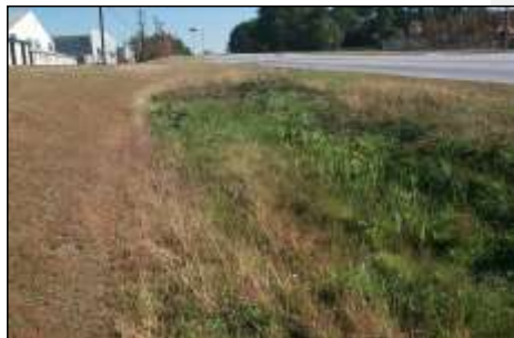
Enhanced Wet Swale
