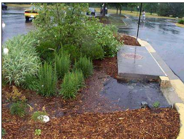
Figure 4.2-4 Bioretention Area After Storm
