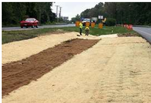
Figure 4.4-4. Linear Bio-swale (Source MDSHA)
