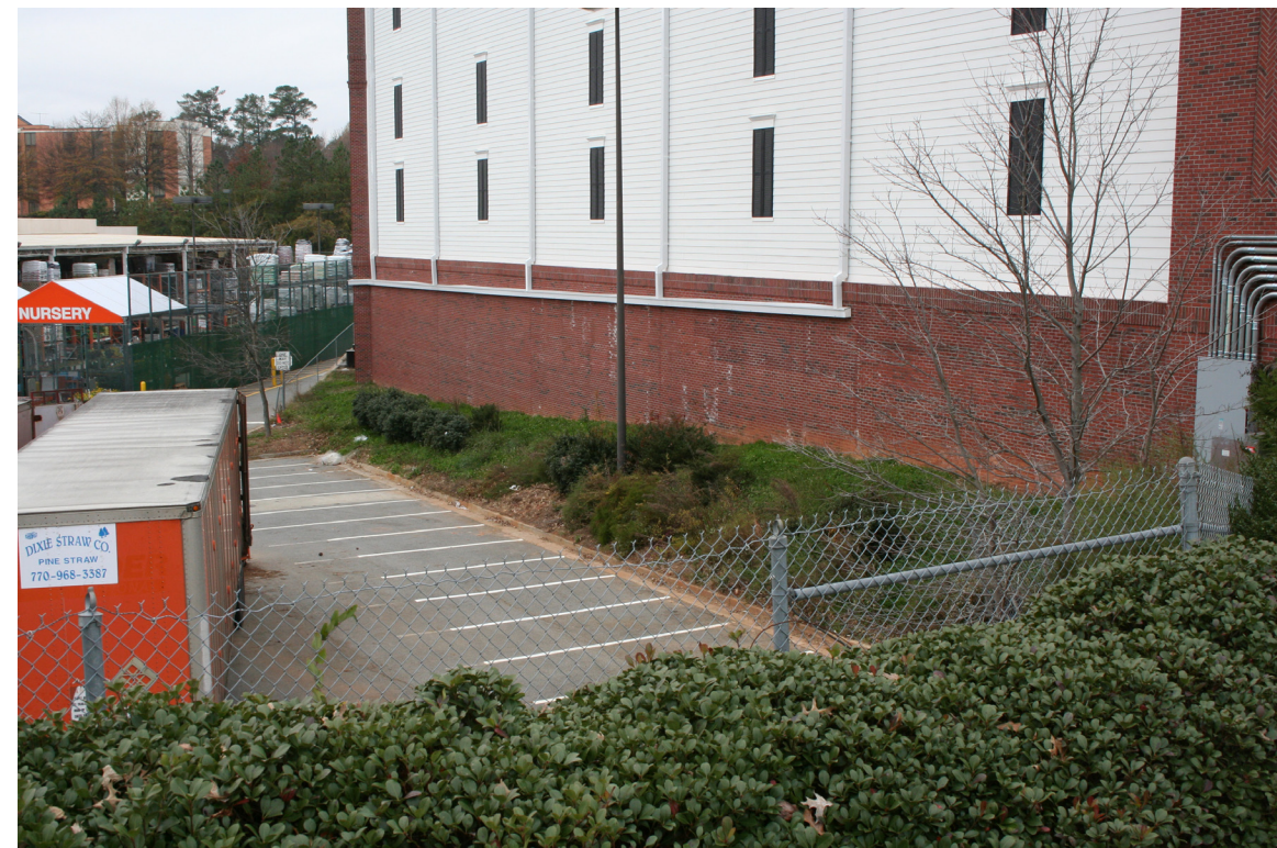
Northeast side of site: topography change of one story from self storage to Home Depot parking
