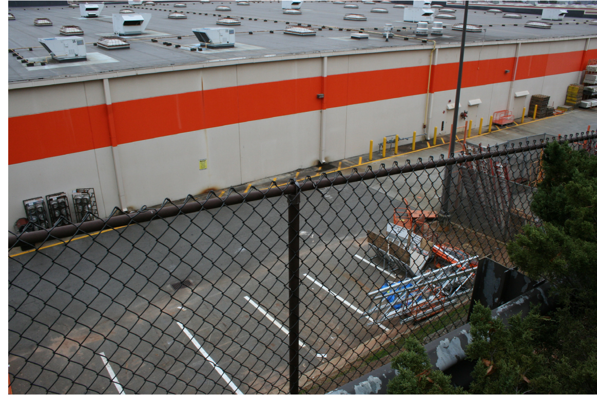
Northwest side of site: severe topography change from road to service entrance
