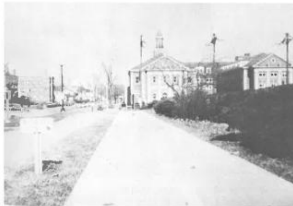
6. A bike track: Improvements within street right-of-way
