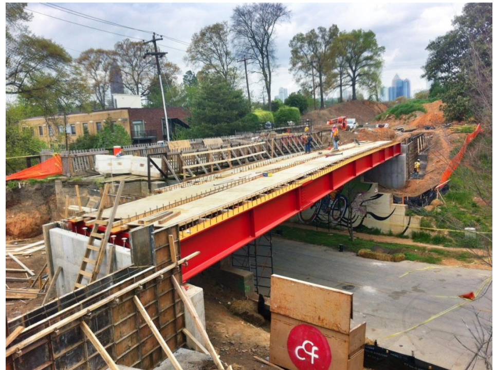
The Atlanta BeltLine Under Construction Over Ralph McGill Boulevard
