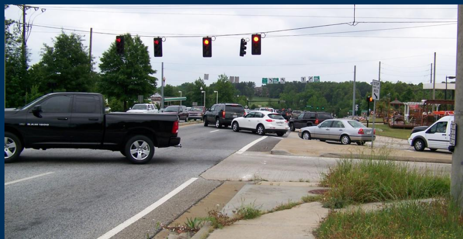
Hamilton Mill Road at I-85
