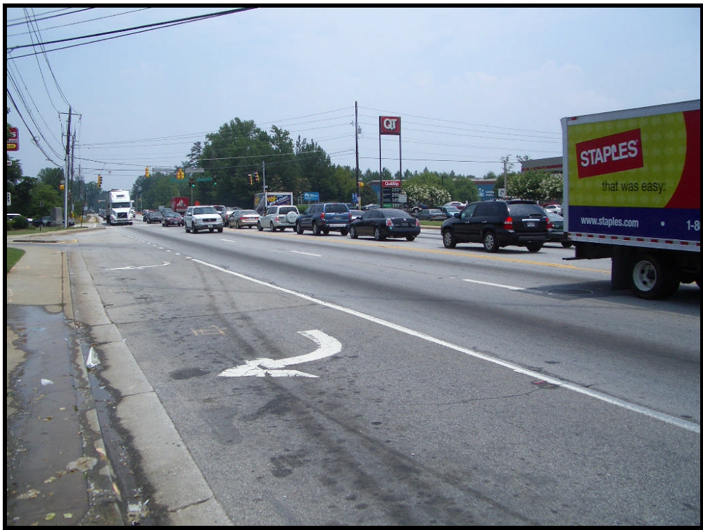
Photograph 10 – Panola Road Facing North Toward Panola Industrial Boulevard
