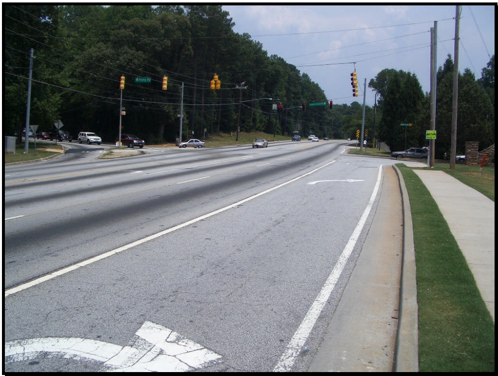
Photograph 5 – Covington Highway Facing East at Young Road
