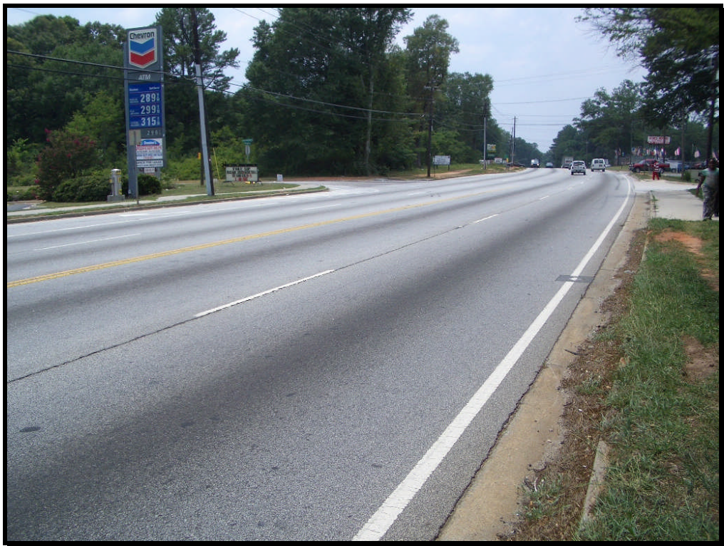
Photograph 3 – Covington Highway Facing West at Park Central Boulevard
