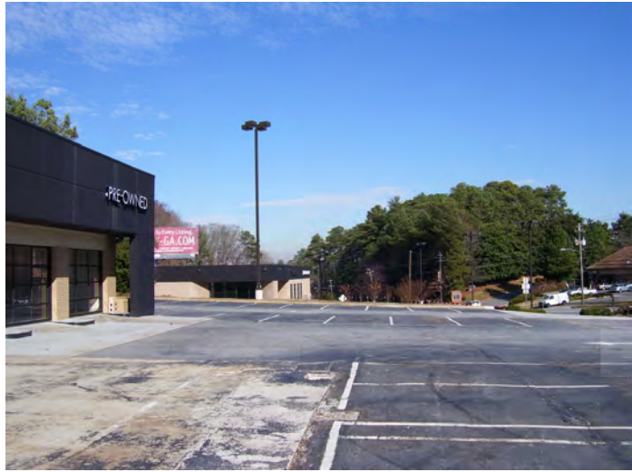
These commercial properties on the northwest corner of Dalrymple Road and Roswell Road are vacant but not abandoned. Such vacant properties are not extensive in Sandy Springs, and prospects for reuse or redevelopment appear promising.
