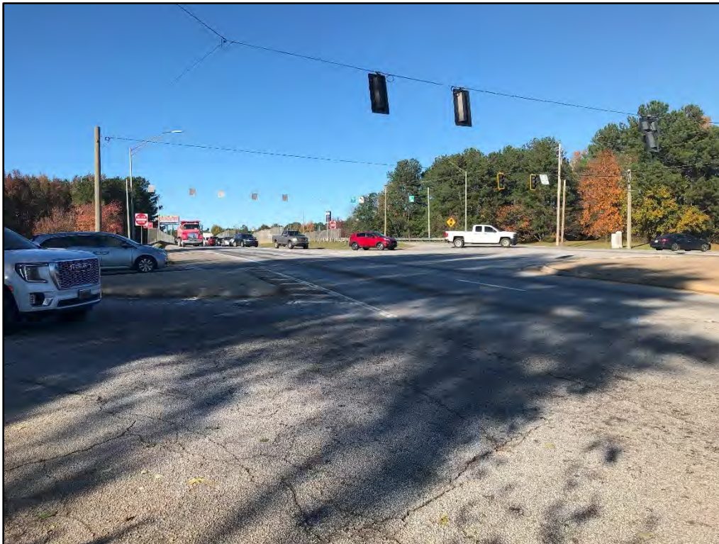
Figure 5: I-85 Northbound Right Turn at SR 74 – Moderate Distress/Cracking
