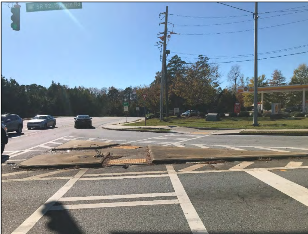
Figure 3: Oakley Industrial Boulevard Right Turn at SR 92 – Slight Distress/Cracking
