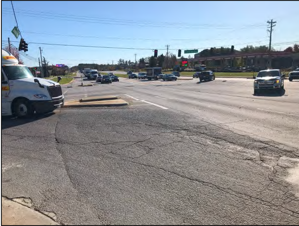
Figure 5: I-85 Northbound Right Turn at SR 74 – Moderate Distress/Cracking
