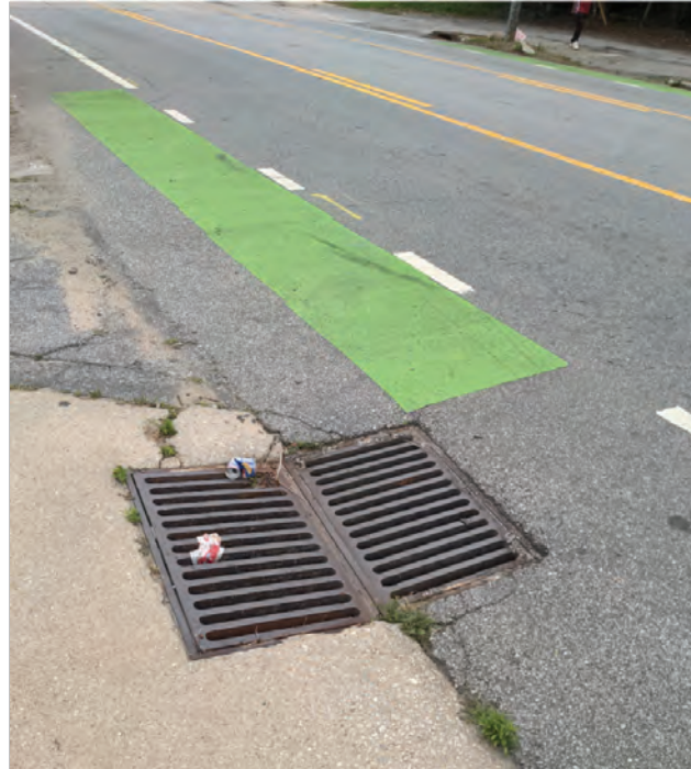
C5. Drain bump hazard and curb cut partially paved over
