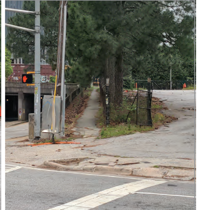
R6. No detectable warning strips at intersection's ramps; no ramps on the southern sidewalk and north-west ramp has large vertical disjoints, cracked concrete, and debris.
