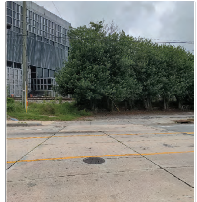
C9. Large curb cut with debris and cracks
