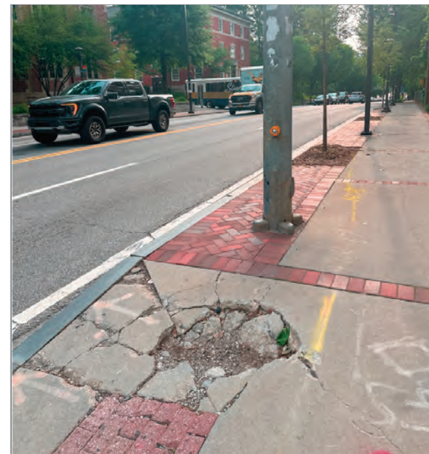
R8. Large cracks in the southeast corner sidewalk near the ramp; creates uneven tripping hazard
