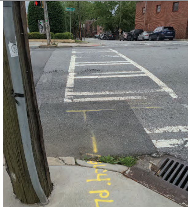
R3. Southwest corner has no ramp and the northeast corner has no southbound ramp. Southeast ramp is poorly aligned
