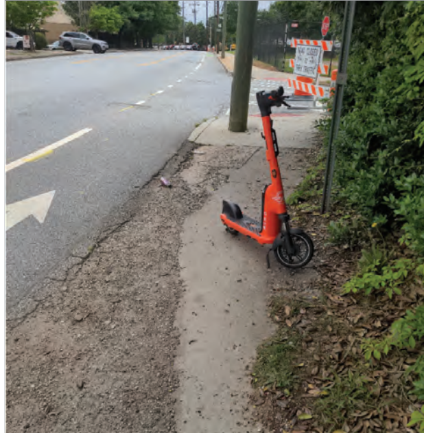
C2. Large curb cut with debris and cracks
