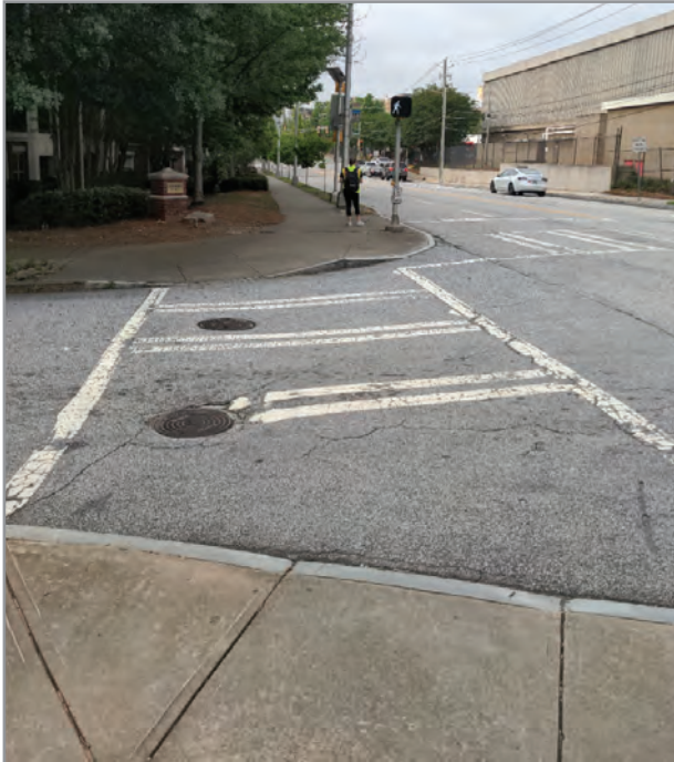
R9. Ramps on east side have no detectable warning strips and are poorly aligned.
