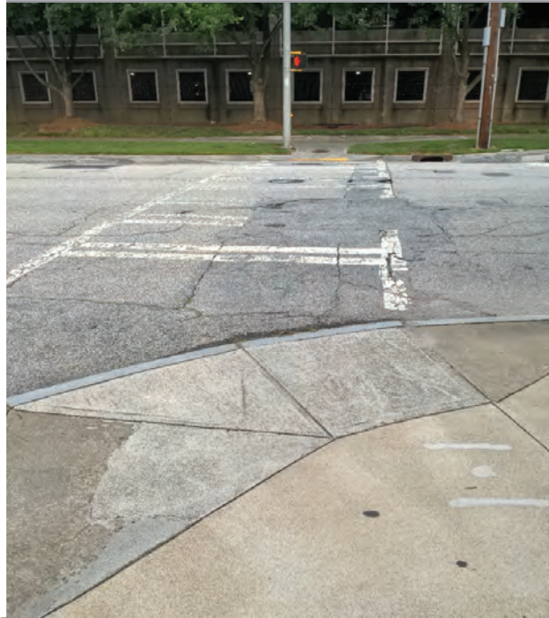
R9. Ramps on east side have no detectable warning strips and are poorly aligned.
