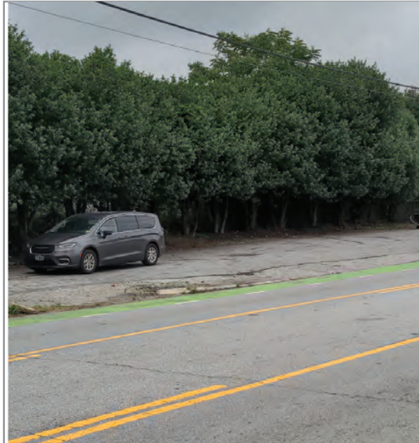
C8. Large curb cut with debris and cracks
