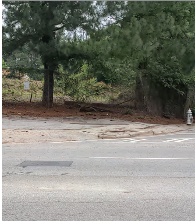
R6. No detectable warning strips at intersection's ramps; no ramps on the southern sidewalk and north-west ramp has large vertical disjoints, cracked concrete, and debris.
