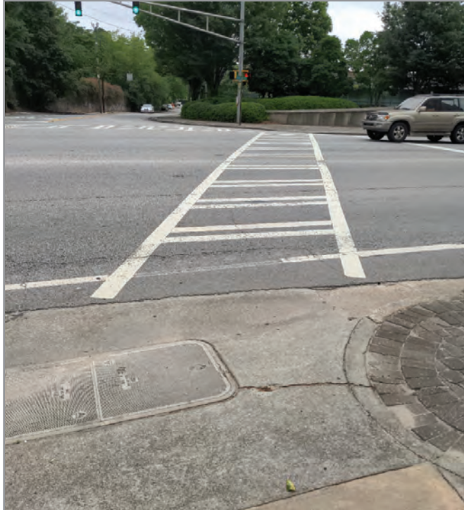
R6. No detectable warning strips at intersection's ramps; no ramps on the southern sidewalk and north-west ramp has large vertical disjoints, cracked concrete, and debris.
