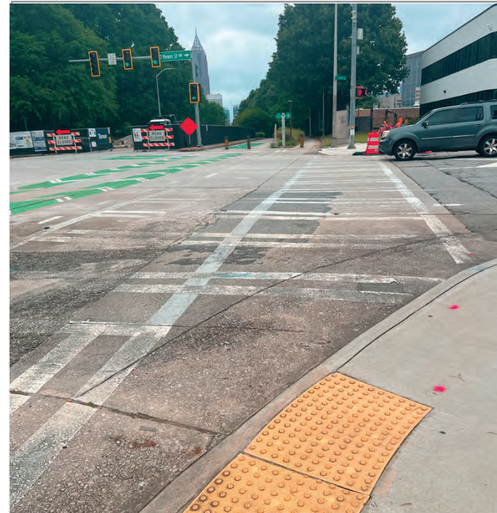
R2. Southeast corner is missing detectable warning strips and southwest corner has poorly aligned ramps
