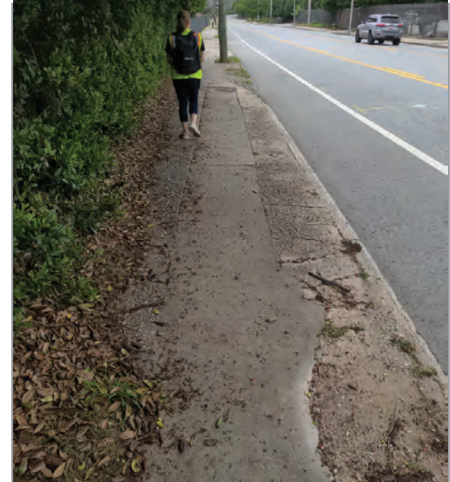
C3. Debris and large curb cut along length
