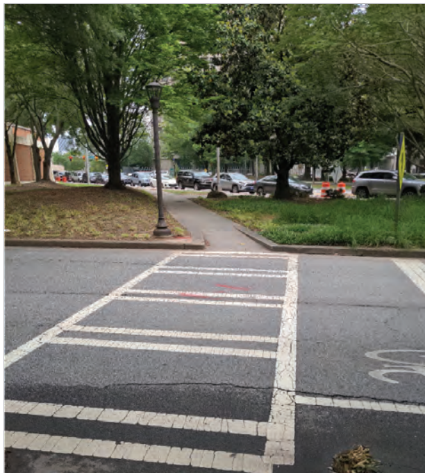
R7. Missing detectable warning strip on southside ramp
