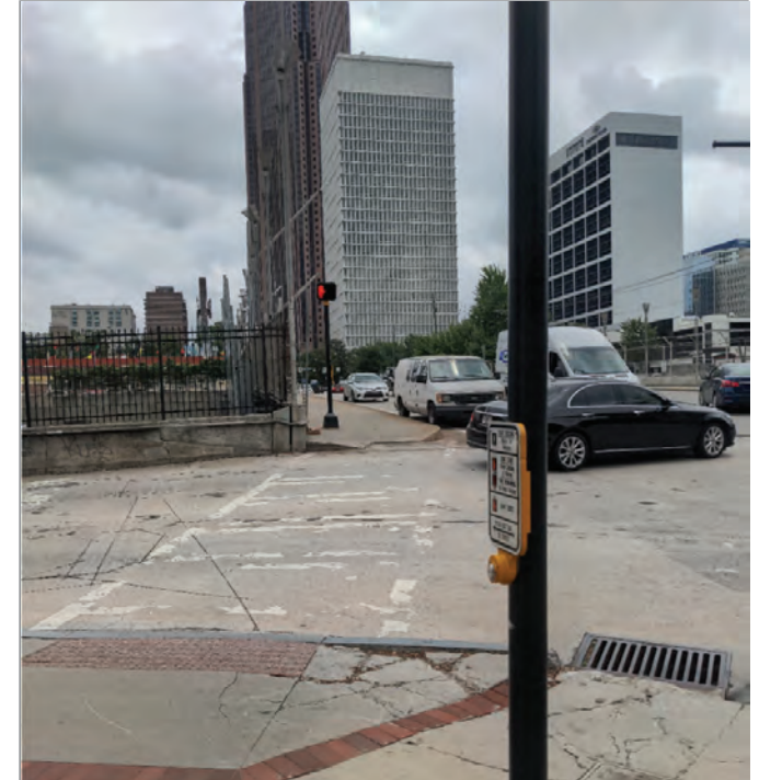
R10. Northeast missing a detectable warning strip/ramp is cracked and not flush with roadway; and the northwest corner has large cracks and uneven concrete
