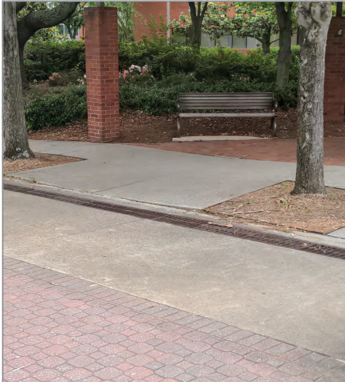
R1. No detectable warning strips at entry to raised crossing
