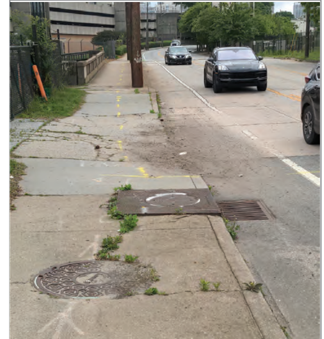
C6. Large curb cut with debris and cracks
