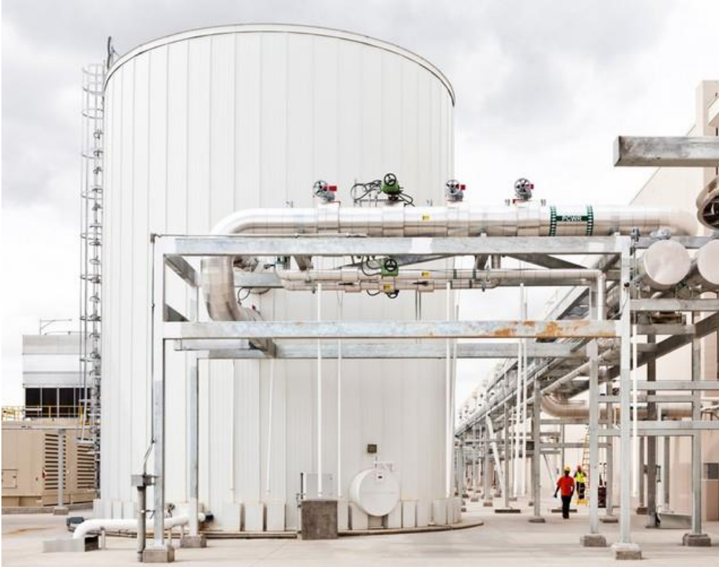
Water tank reservoir for cooling the servers and buildings.
