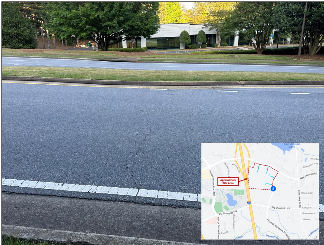
Figure 5: Chastain Meadows Parkway Southbound Turn Lane Minor Cracking
