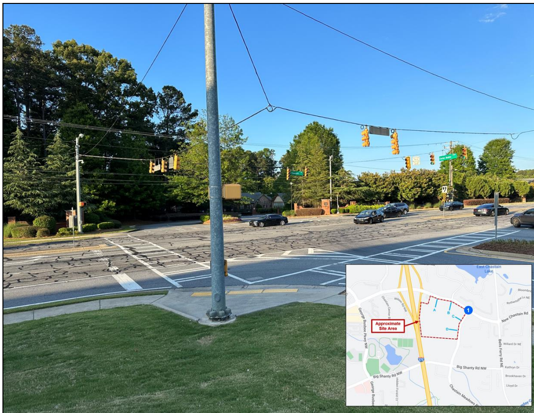
Figure 4: Chastain Road Repaired Pavement Cracking
