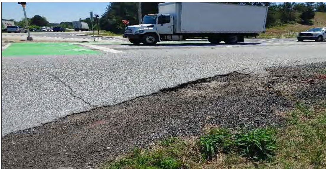
Figure 19: Thornton Road (SR 6) at Riverside Parkway Southbound Right – Degraded Shoulder
