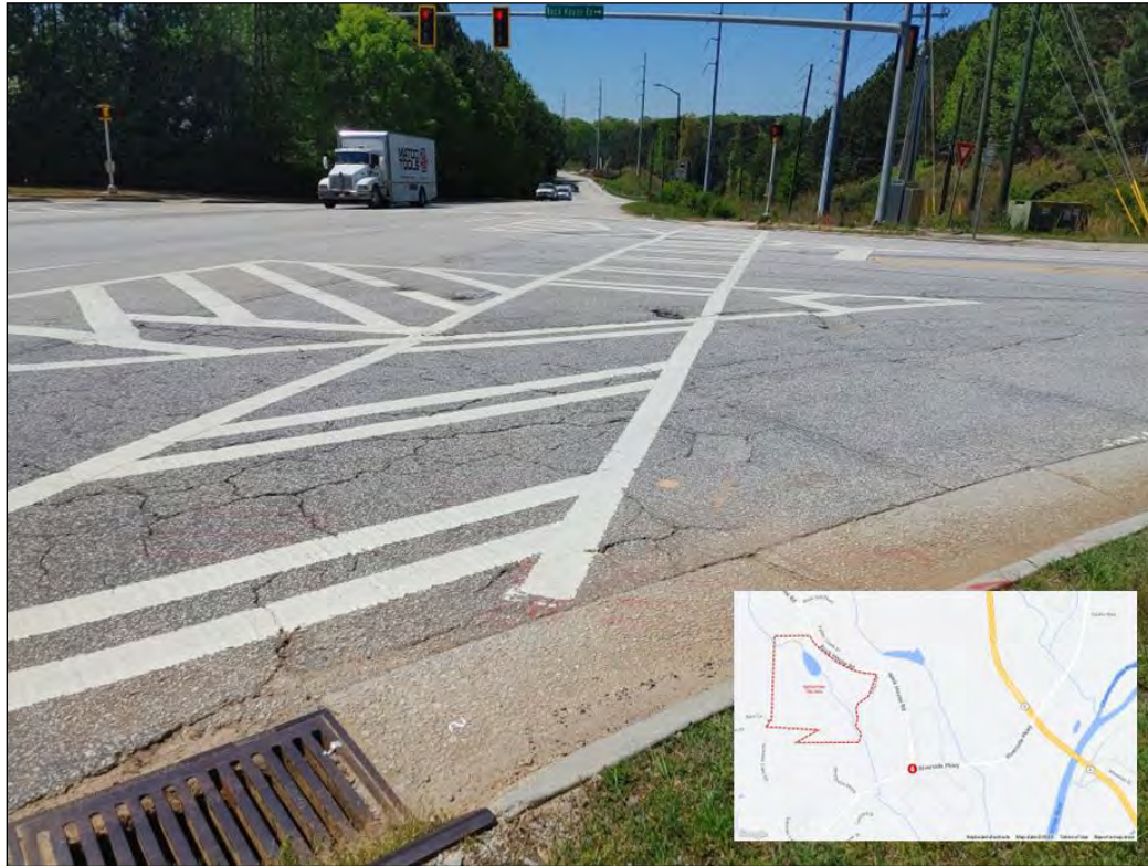
Figure 11: Westbound Riverside Parkway at Rock House Road Potholing and Cracking
