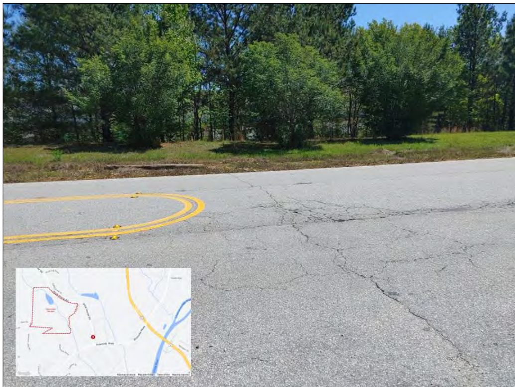
Figure 8: Southbound Rock House Road Cracking
