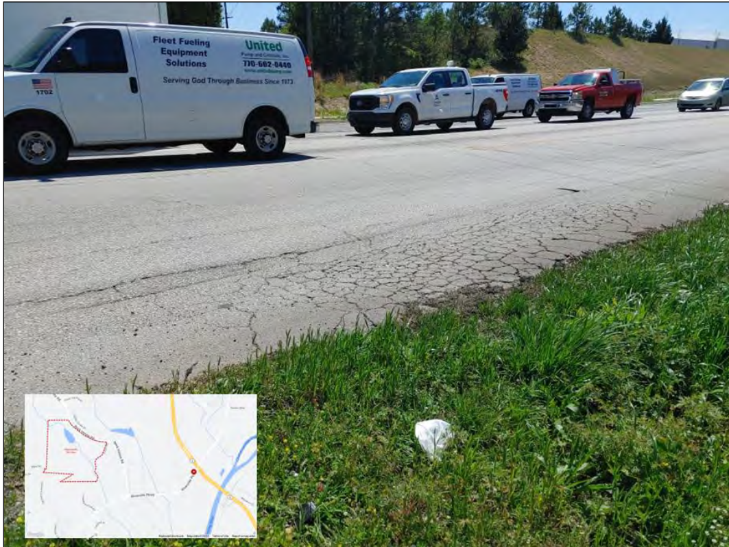
Figure 17: Westbound Riverside Parkway Cracking
