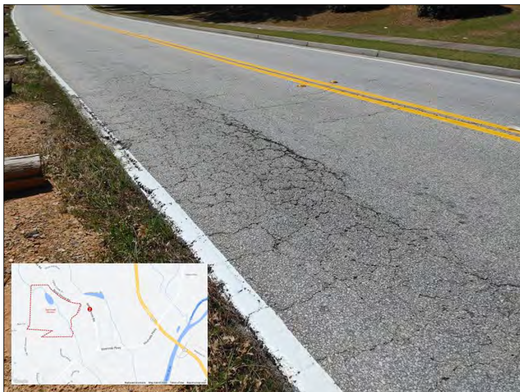
Figure 6: Southbound Rock House Road Cracking
