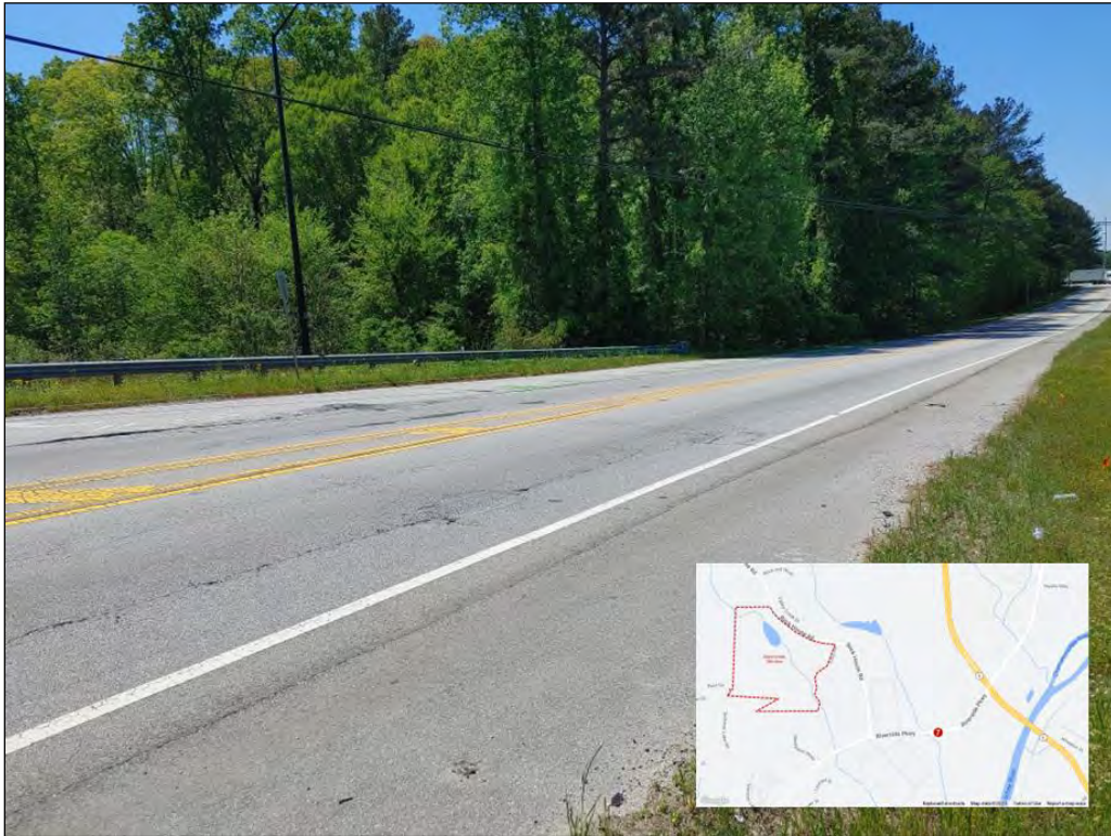
Figure 13: Westbound Riverside Parkway Potholing and Cracking
