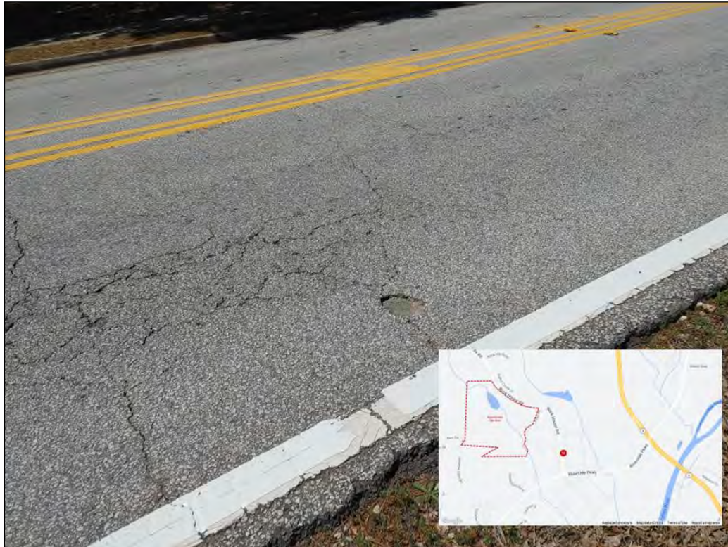
Figure 7: Northbound Rock House Road Potholing
