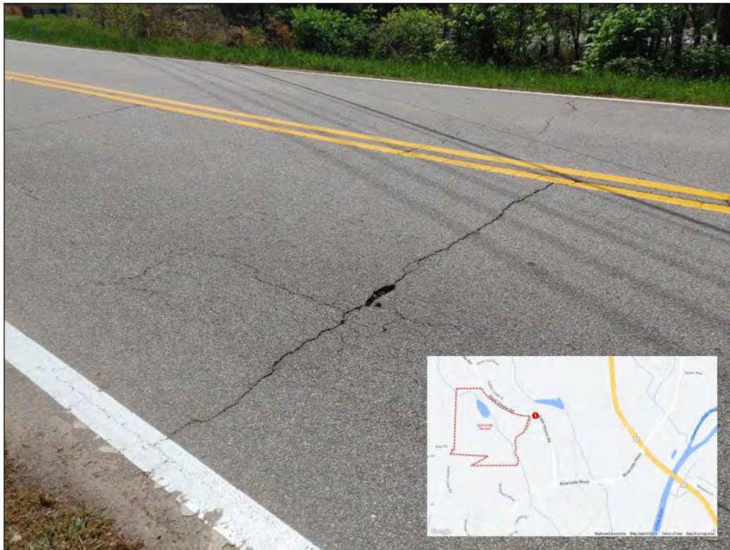
Figure 5: Northbound Rock House Road Potholing
