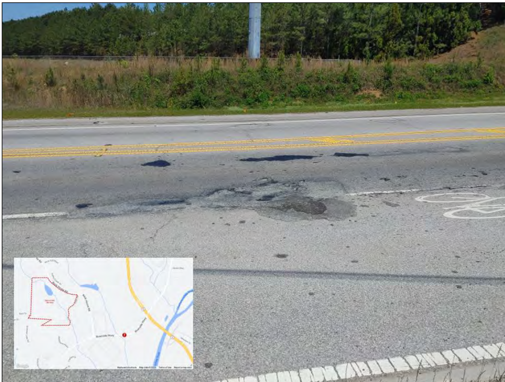
Figure 12: Eastbound Riverside Parkway Potholing
