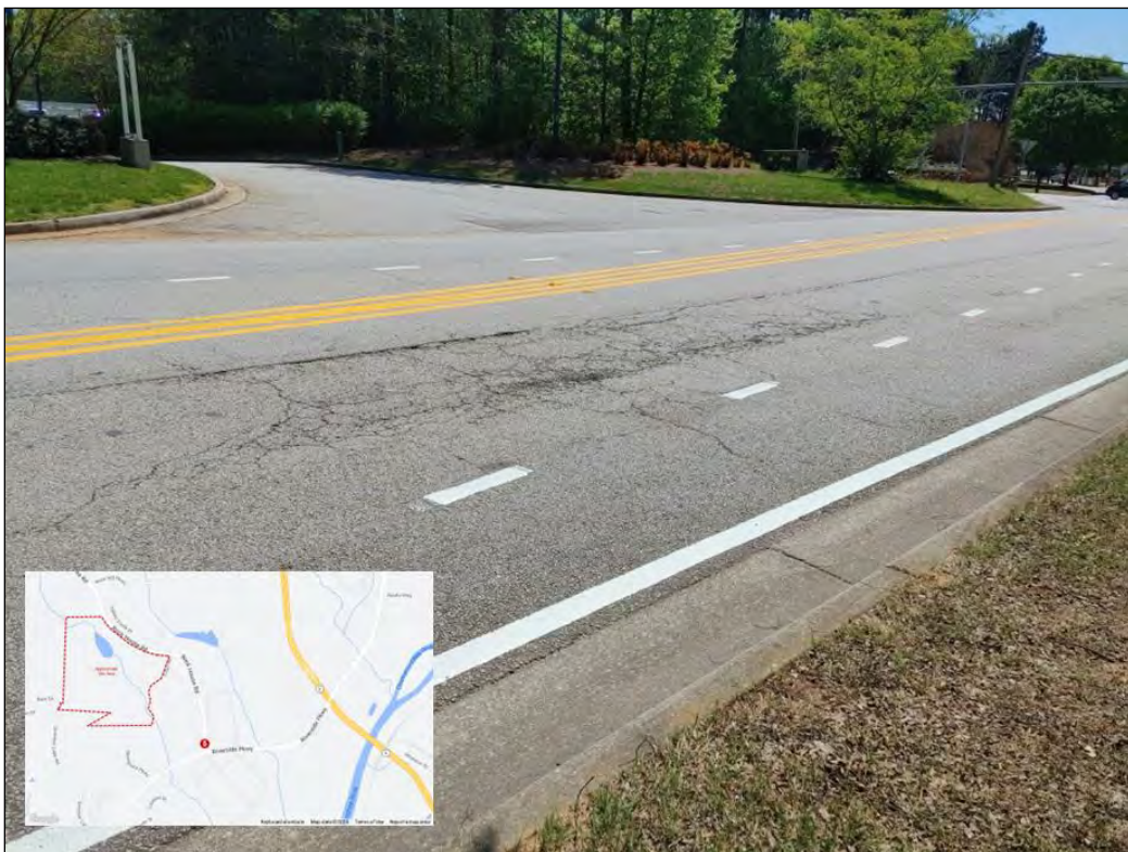
Figure 10: Southbound Rock House Road Cracking
