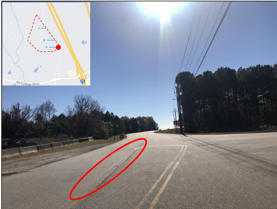
Figure 5: Southbound Price Drive Minor Pavement Cracking
