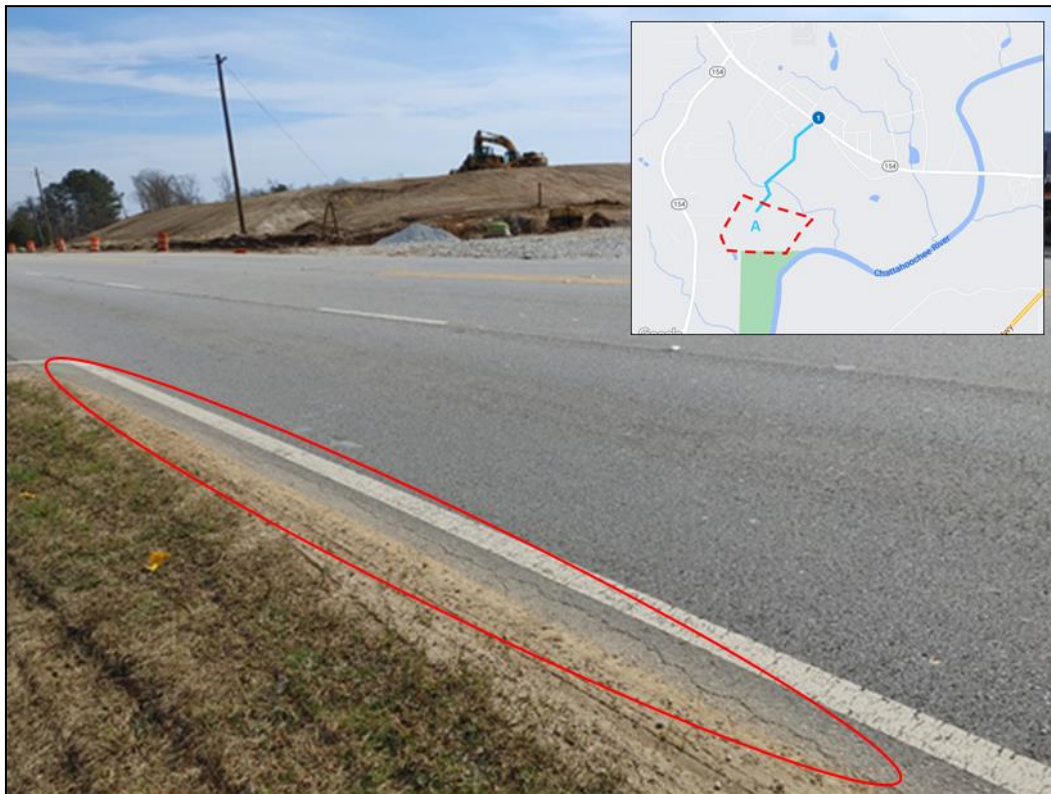
Figure 4: Westbound Fairburn Road (SR 70/SR 154/SR 166) Minor Shoulder/Pavement Cracking
