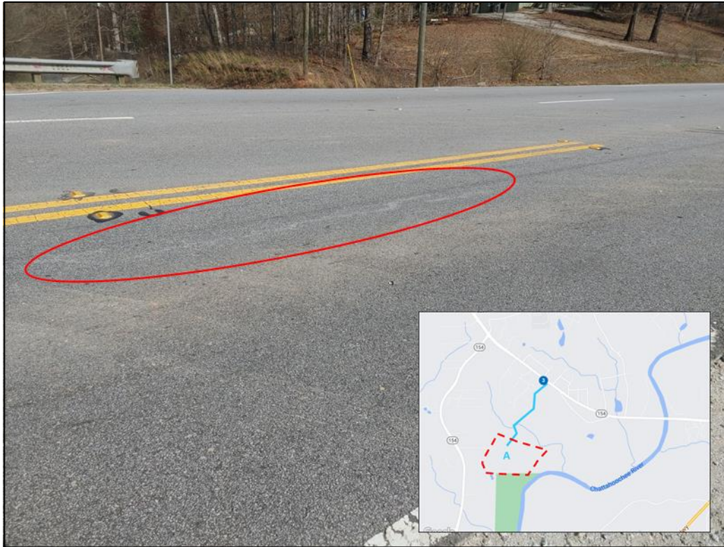
Figure 5: Eastbound Fairburn Road (SR 70/SR 154/SR 166) Minor Pavement Cracking
