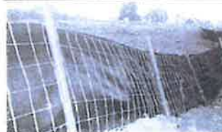
Figure 5. Typical Type "C" Silt Fence
