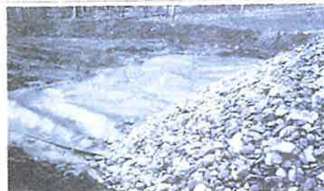
Figure 2. Geotextile Underliner Under Gravel Pad
