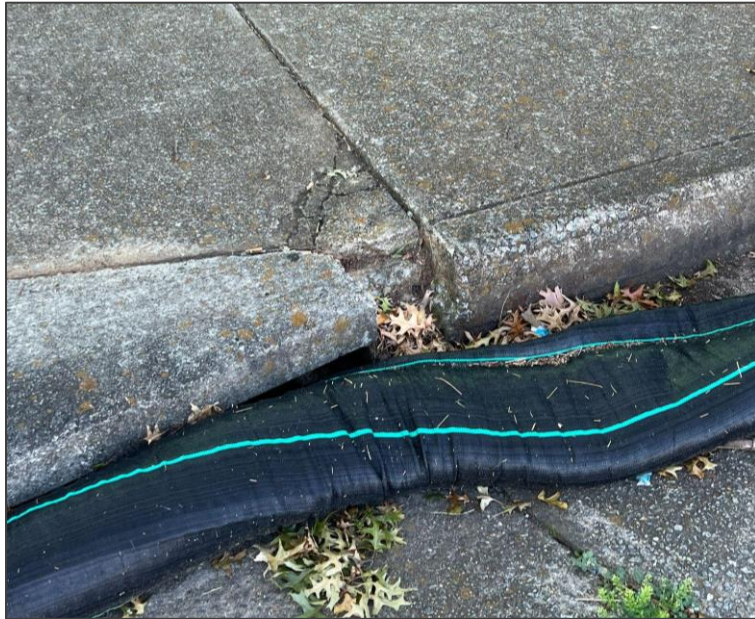
Figure 9: Minor Curb Cracking along Murphy Avenue
