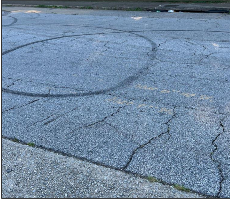
Figure 3: Murphy Avenue Pavement Cracking
