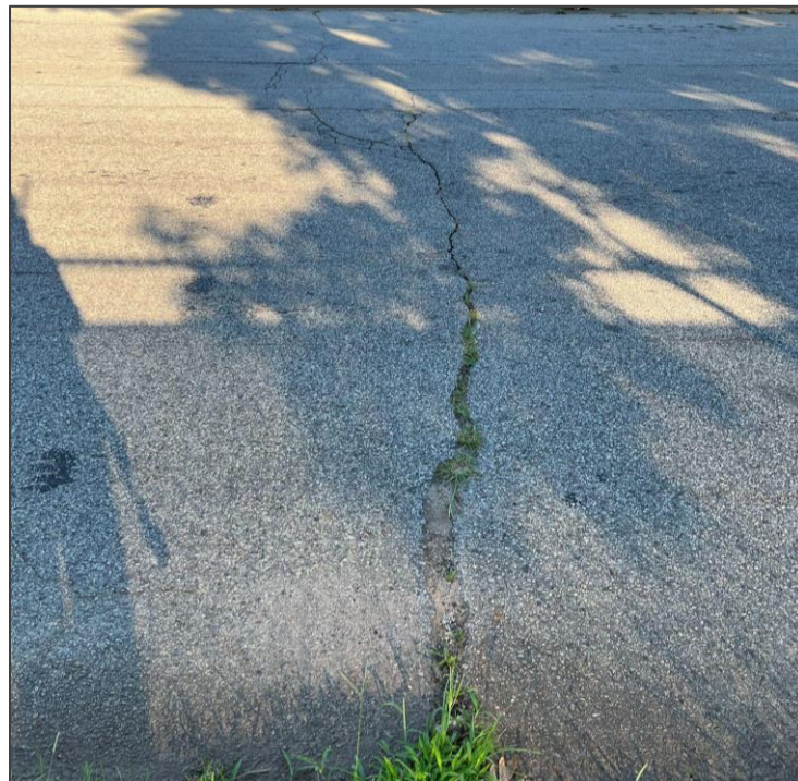
Figure 4: Murphy Avenue Pavement Cracking
