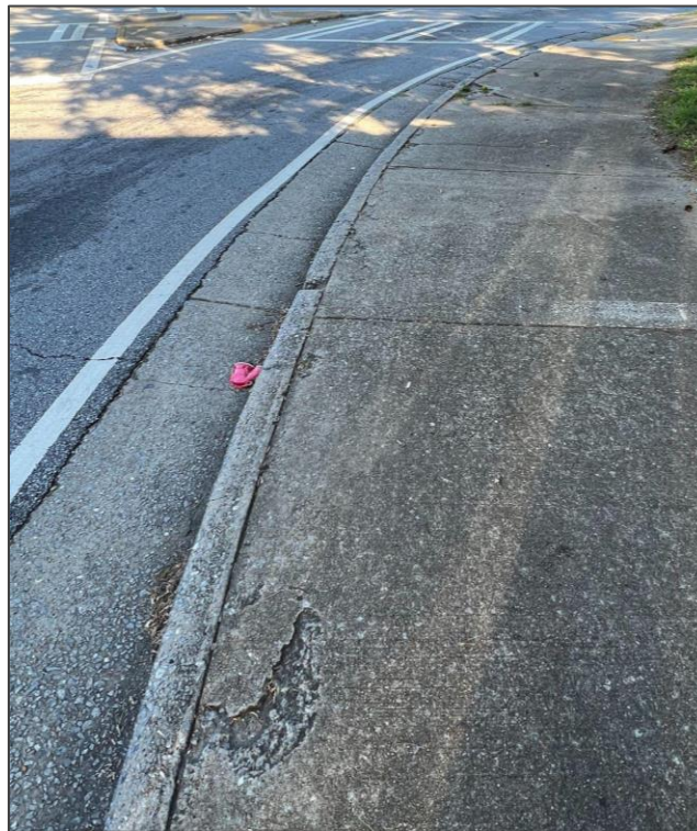
Figure 10: Minor Curb Cracking along Dill Avenue at Lee Street (US 29/SR 14/SR 139/SR 154)
