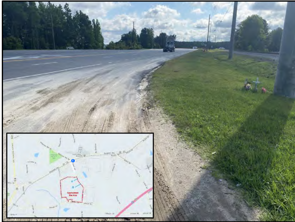
Figure 4: Roosevelt Highway (US 29/SR 14) Minor Rutting of the Pavement
