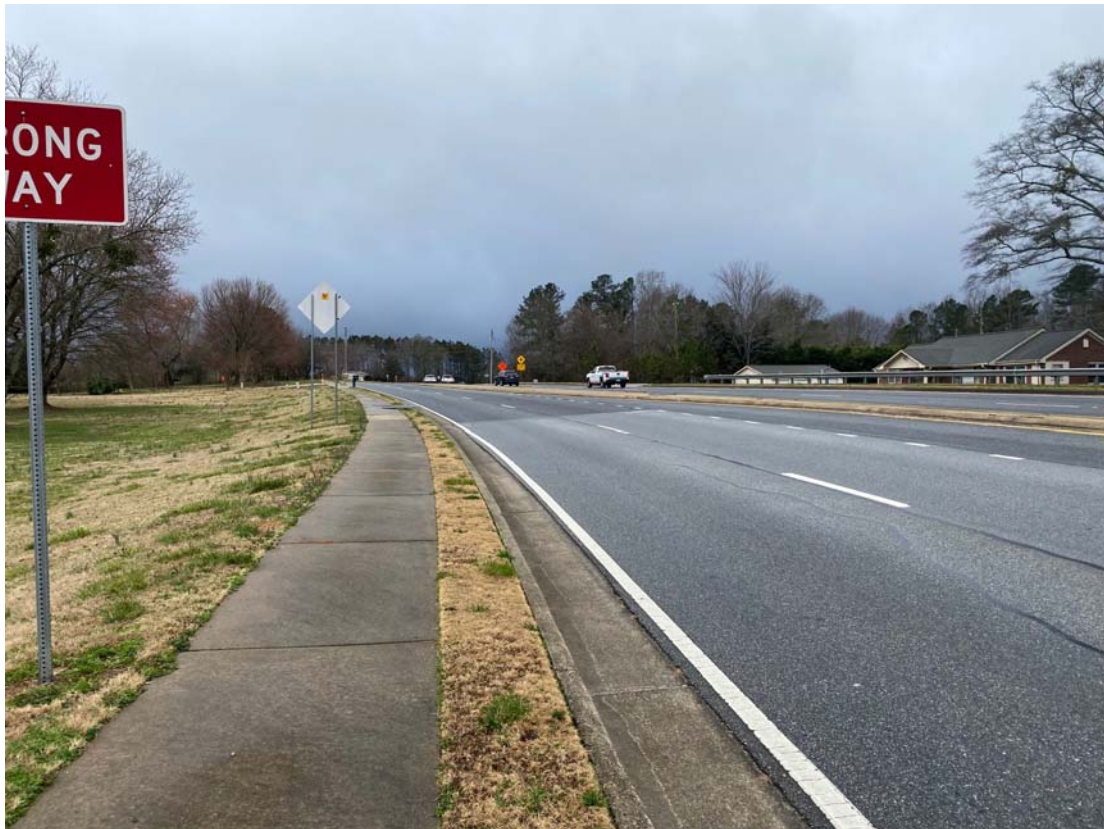
Gravel Springs Road at Proposed West Driveway Pavement in good condition
