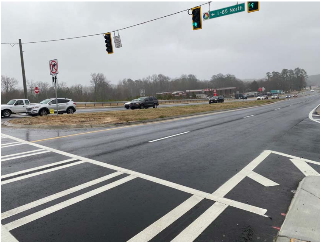
Gravel Springs Road at I-85 on ramp Pavement newly installed and shows no signs of issue
