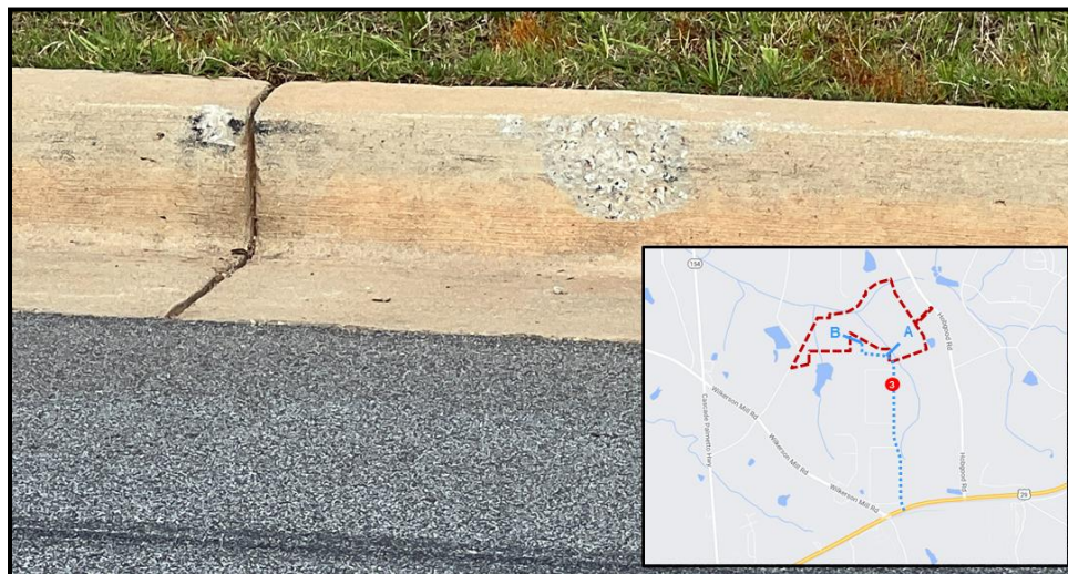
Figure 6: Palmetto Logistics Parkway Minor Curb Cracking
