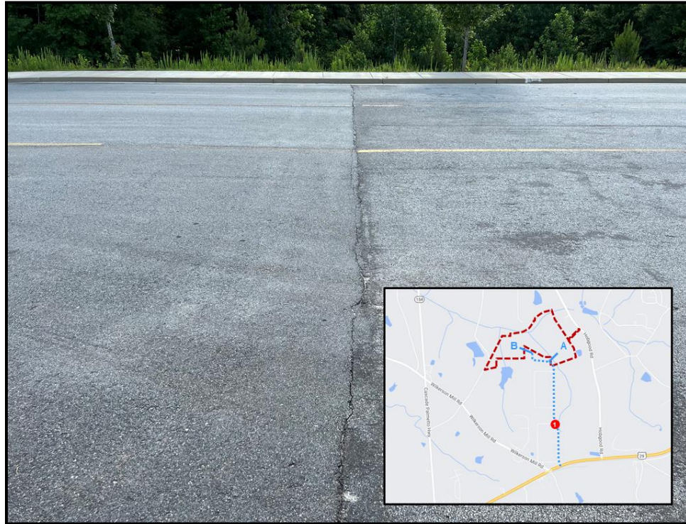
Figure 4: Palmetto Logistics Parkway Minor Pavement Cracking
