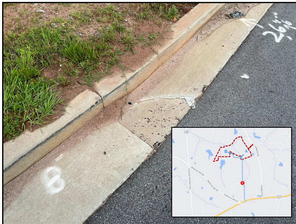
Figure 5: Palmetto Logistics Parkway Minor Curb Cracking
