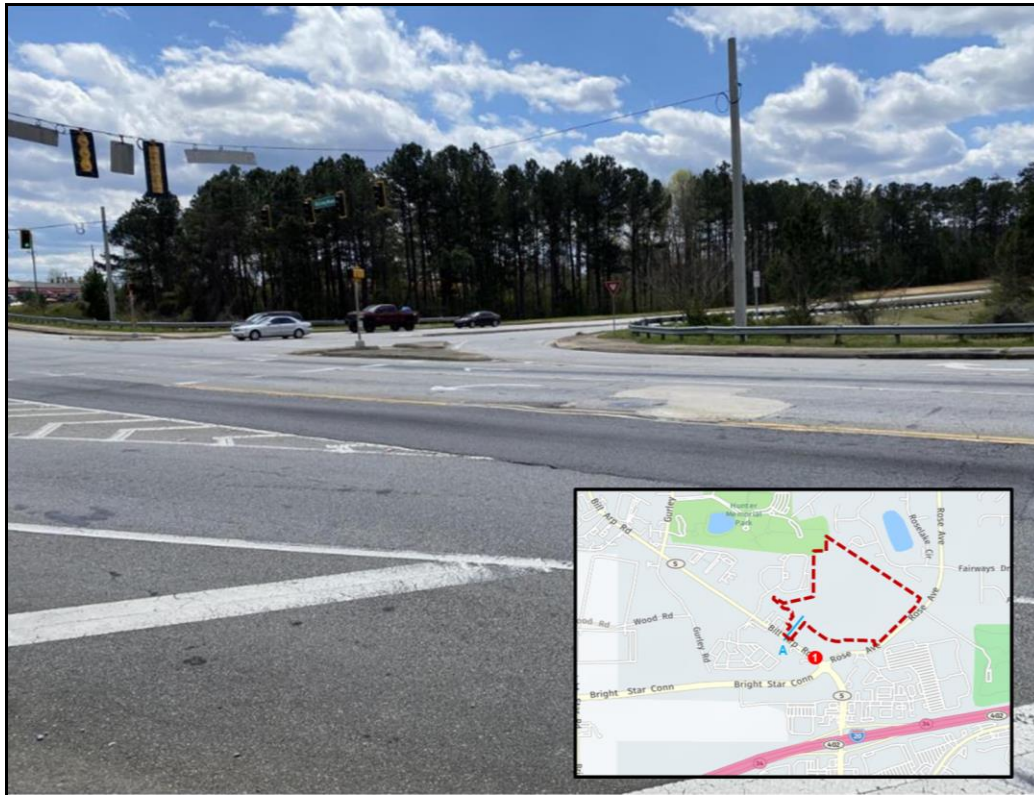
Figure 4: Southbound Bill Arp Road (SR 5) Pavement Warping
