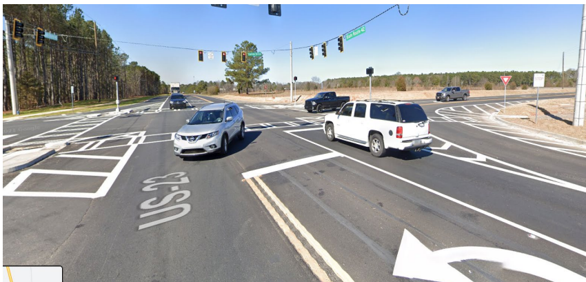
New pavement on intersection of Colvin Drive and SR-42.
