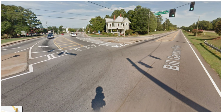
Pavement in good conditions at left turn at the cross-section between Bill Gardner Parkway and SR-42.
