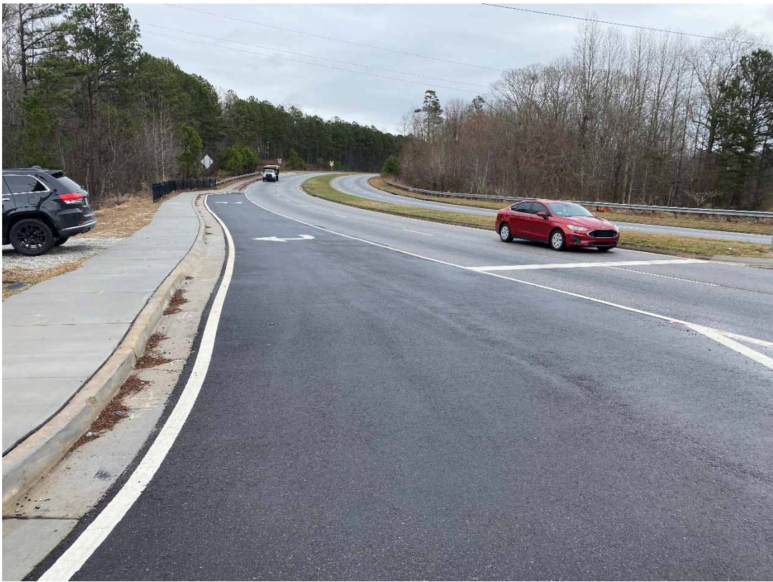
Lithonia Industrial Blvd at Rogers Lake Road Pavement in Good Condition and shows no signs of issue
