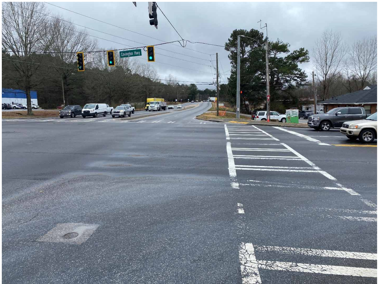
Lithonia Industrial Blvd at Covington Highway Pavement in Good Condition and shows no signs of issue
