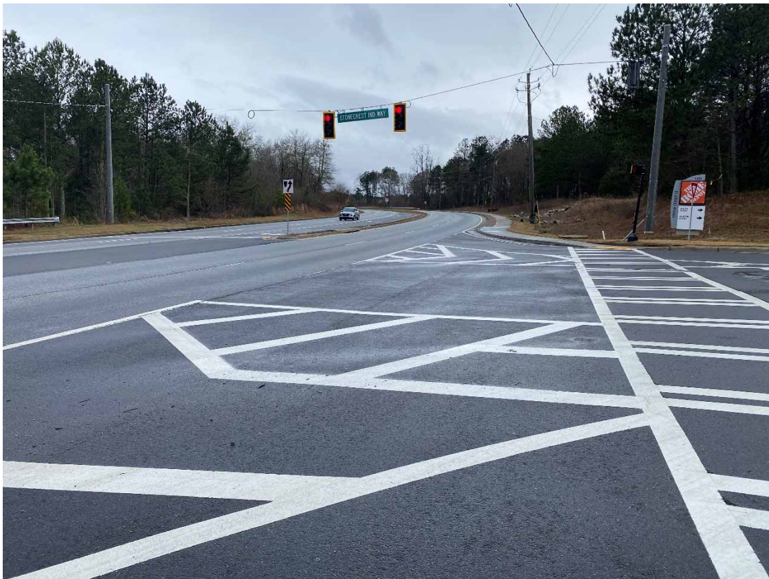
Lithonia Industrial Blvd at Stonecrest Industrial Way Pavement in Good Condition and shows no signs of issue
