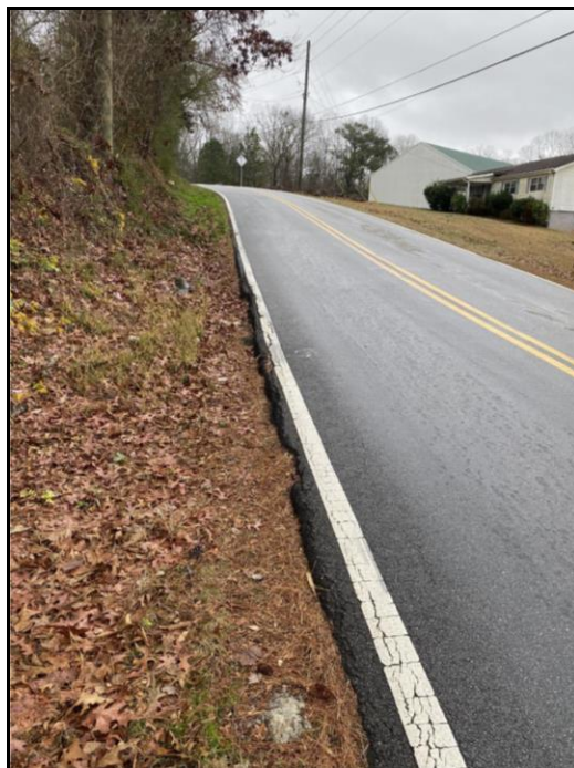
Figure 11: Factory Shoals Road at Douglas Hill Road – Loosened Shoulder
