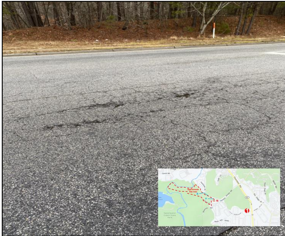
Figure 4: Eastbound Douglas Hills Road Potholing
