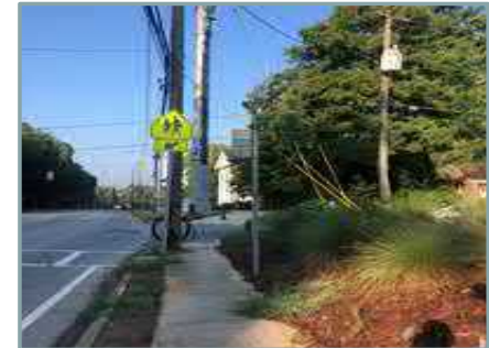
MARTA Stop 901840 along N Decatur Road at Ridgewood Drive. Missing a landing pad.
