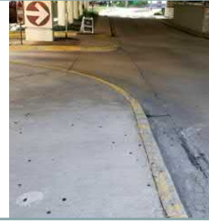
Sidewalk along Lowergate Drive is missing pedestrian ramps at curb cuts.
