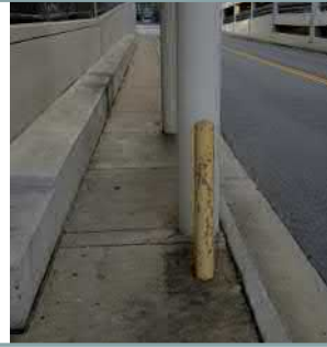
Sidewalk along Gambrell Drive south of Lowergate Garage is impeded by pillar.
