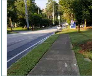
MARTA Stop 901842 along N Decatur Road at Healthgate Drive. No ramp from sidewalk/stop to roadway. Opportunity to tie in bus stop with PATH.
