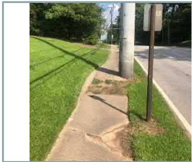
Sidewalk along N Decatur Road east of Westminster Way is in poor condition.
