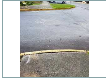
Sidewalk along eastern side of Haygood Drive crossing school driveway. No ramp or crosswalk.
