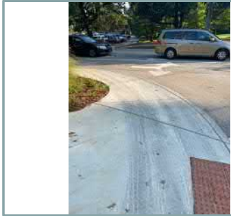
Northwest corner of the intersection of Haygood Drive with N Decatur Road. Tire tracks from wide turning vehicles/ driving on the sidewalk.
