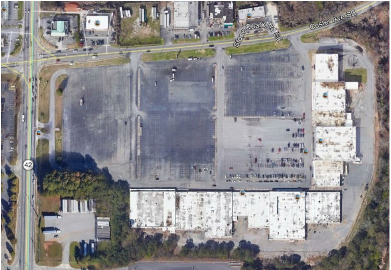
Figure 6: Existing Aerial of Proposed Development
