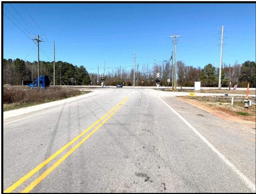
Photograph 7 – Tatum Road Facing North at Railroad Crossing and US 29
