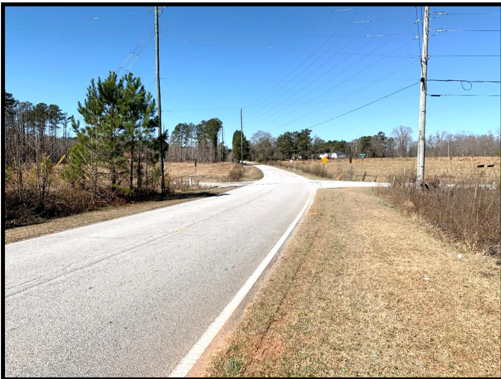
Photograph 9 – Wilkerson Mill Road Facing North at Ono Road
