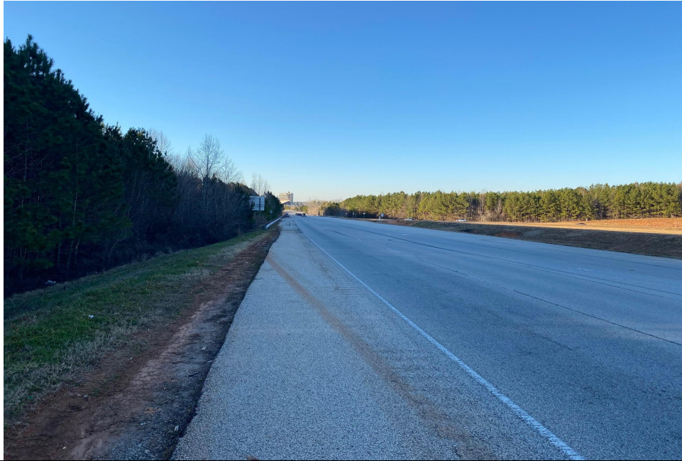
Comments: Site Driveway B looking north.
