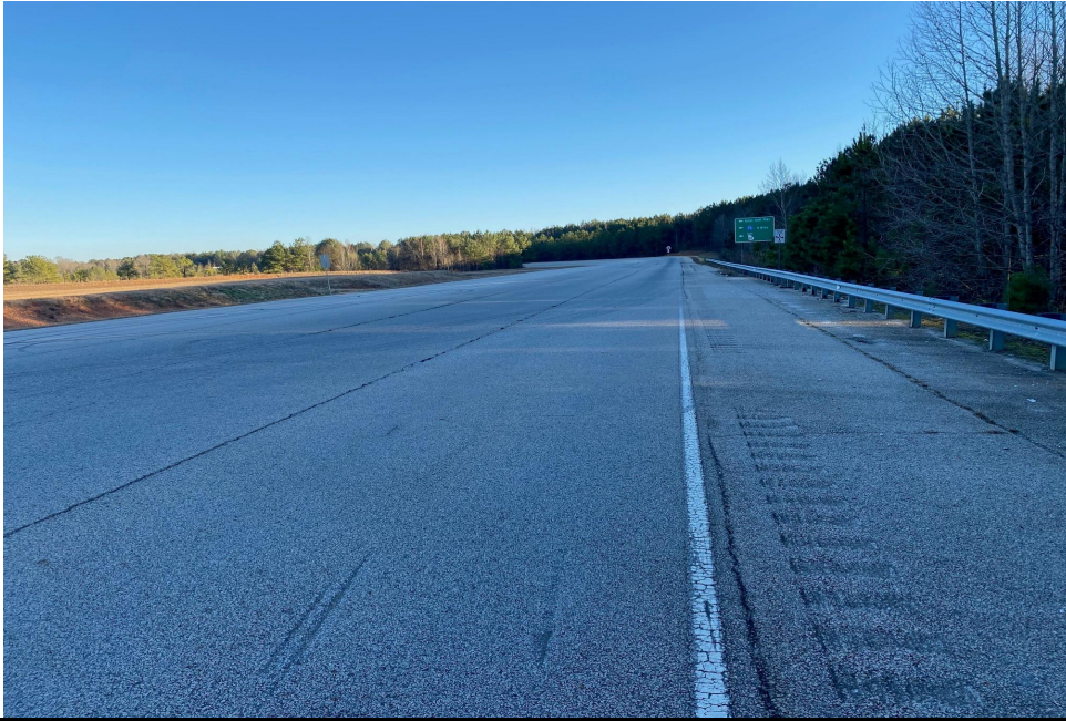
Comments: Site Driveway A looking south.
