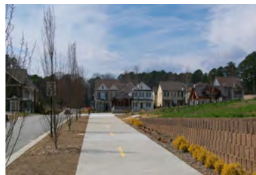
▲ New multi-use trail at Project Renaissance
