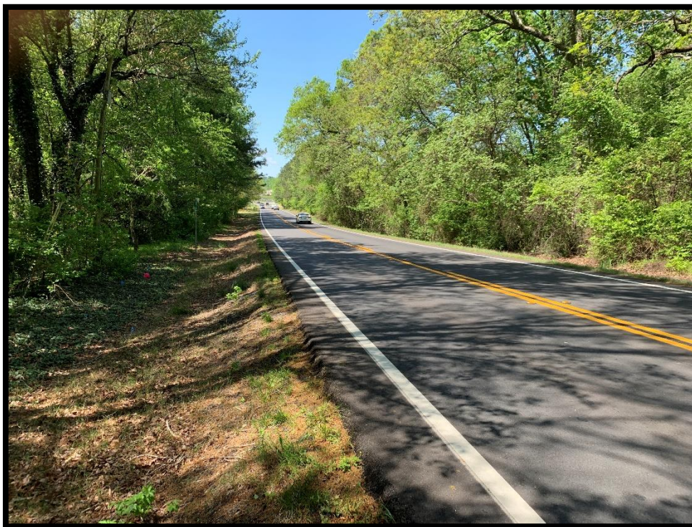
Figure 3 – Photograph of GA 124 Facing West, West of Huntington Hill Trace
