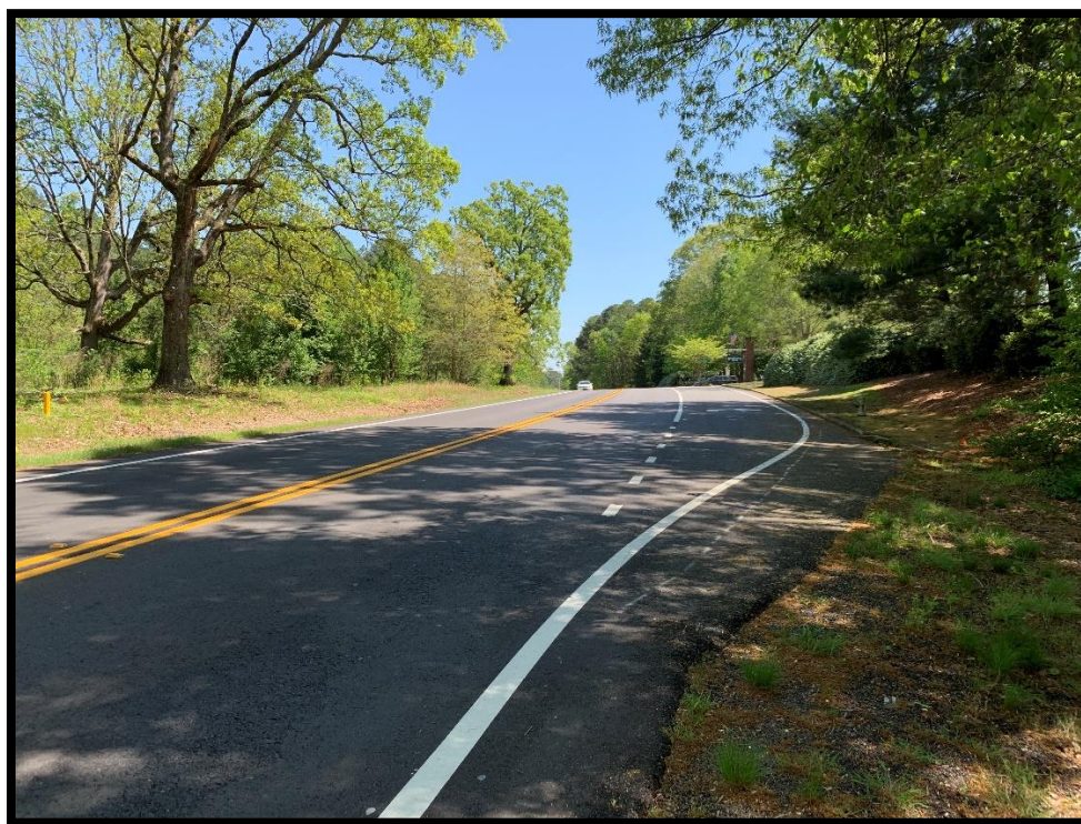
Figure 4 – Photograph of GA 124 Facing East at Huntington Hill Trace
