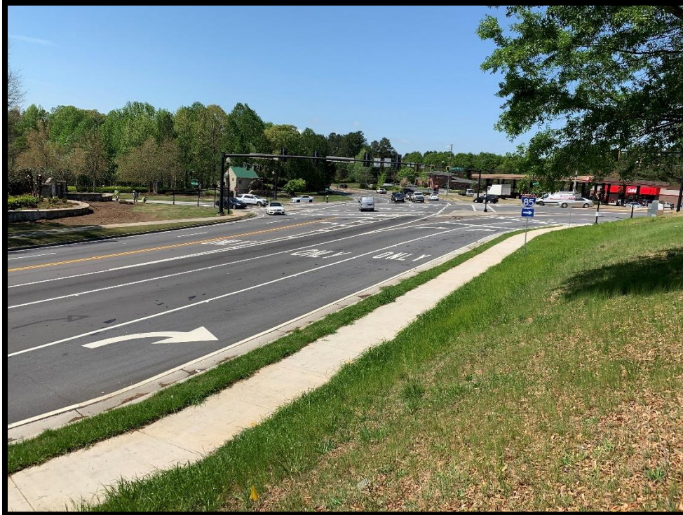
Photograph 1 – GA 124 Facing West at Hamilton Mill Road
