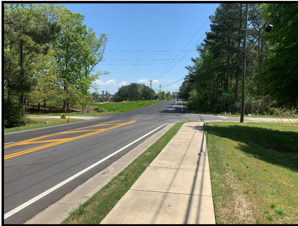
Photograph 8 – GA 124 Facing East at Holman Road
