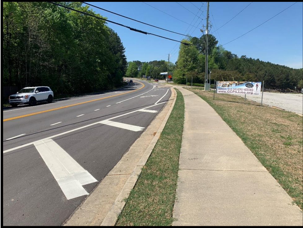
Photograph 9 – GA 124 Facing West Toward Mill Creek HS Right-In / Right-Out Access
