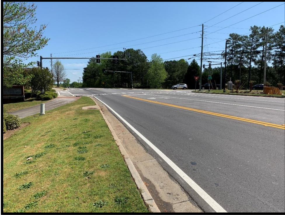
Photograph 3 – GA 124 Facing East at Pine Road
