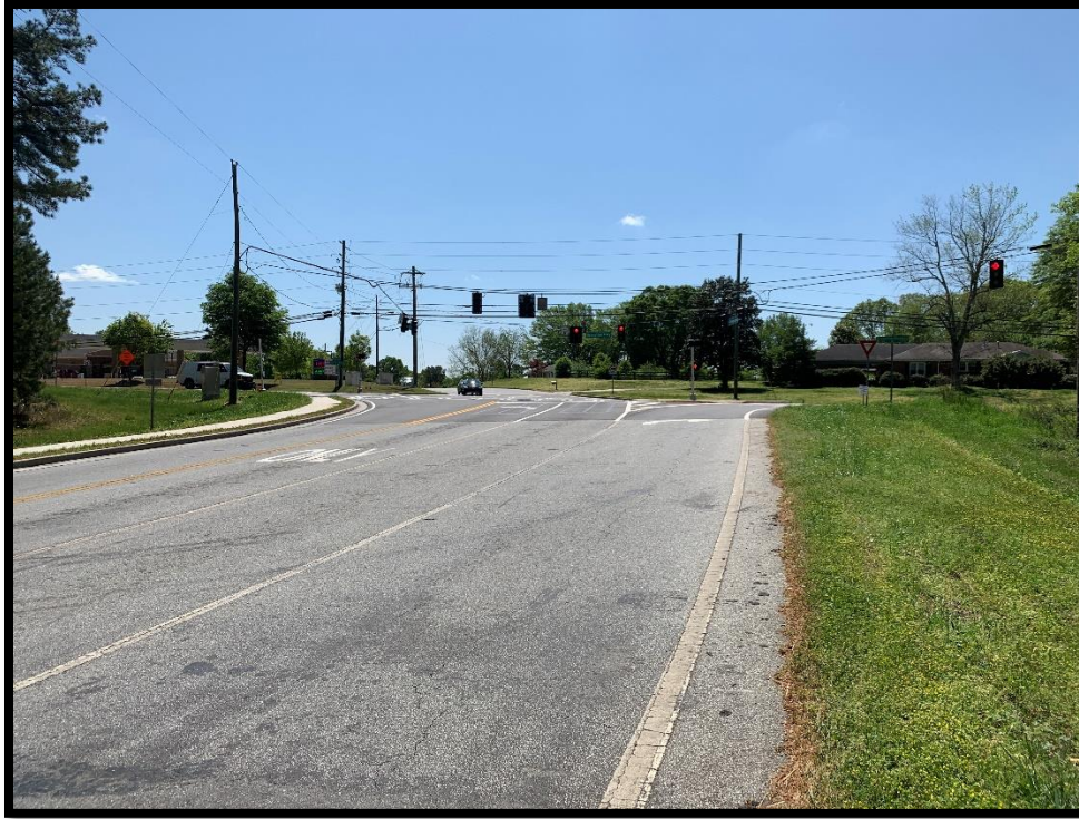
Photograph 7 – Spout Springs Road Facing South at GA 124
