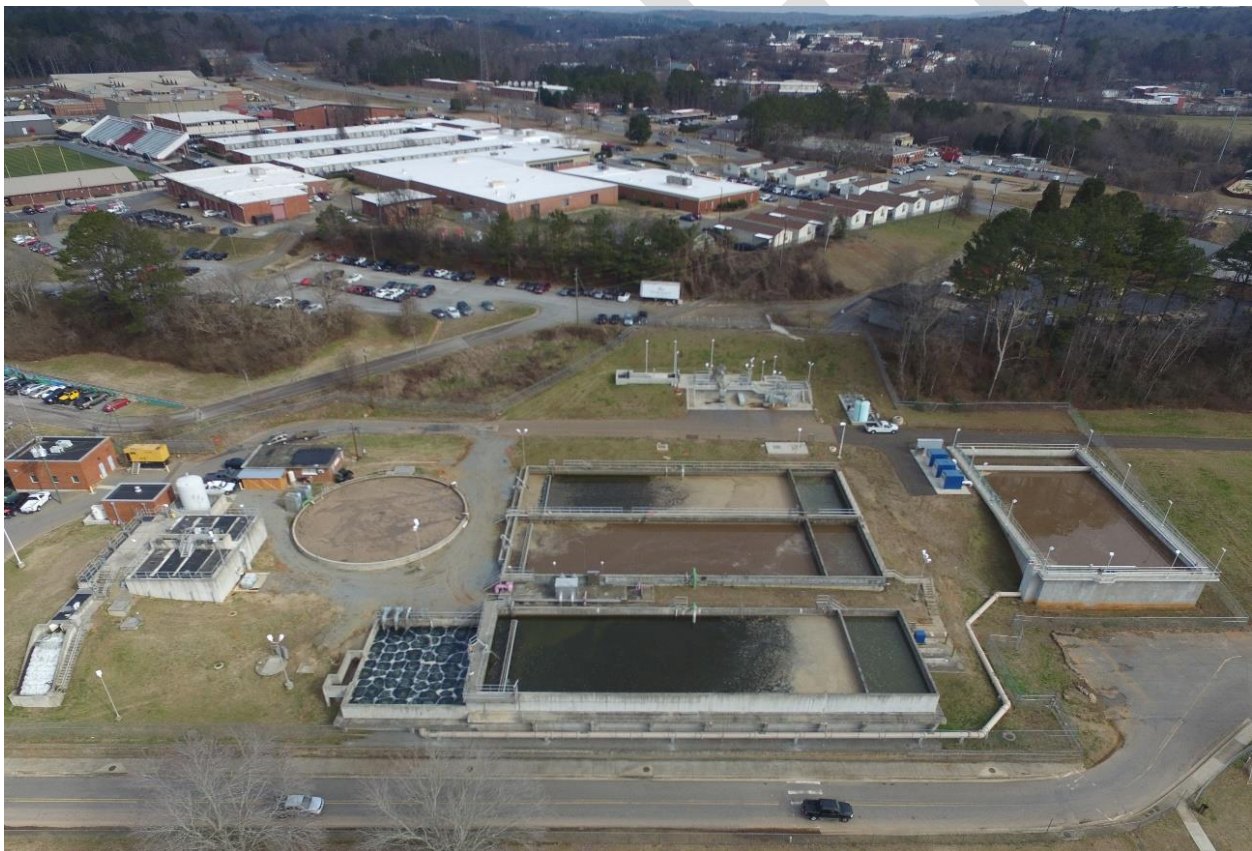
Canton Wastewater Treatment Plant
