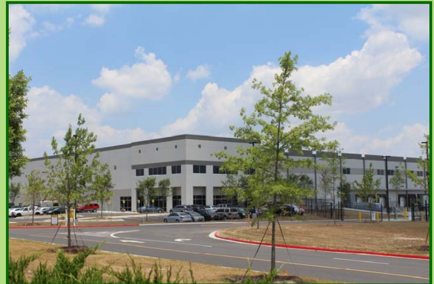
Atlanta Metro Studios / Colliers International—distribution facility.
