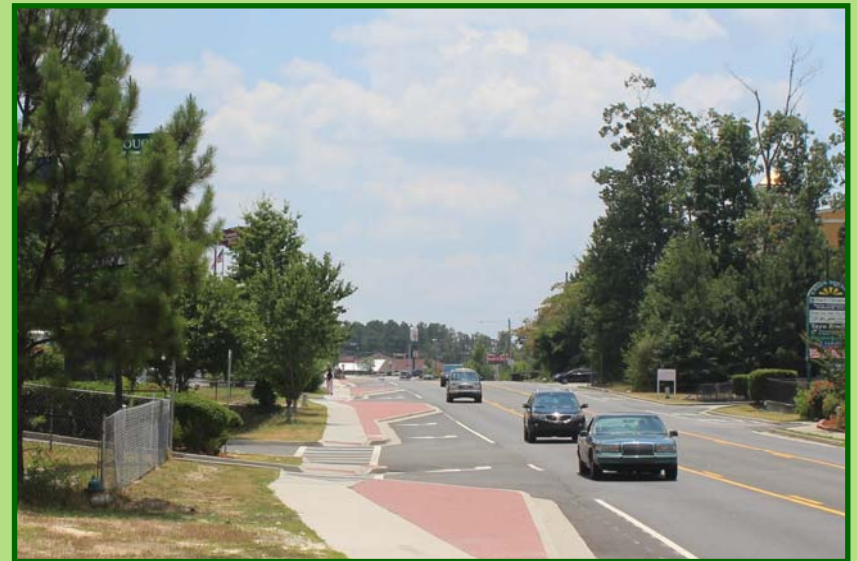
New sidewalks along Shannon Parkway
