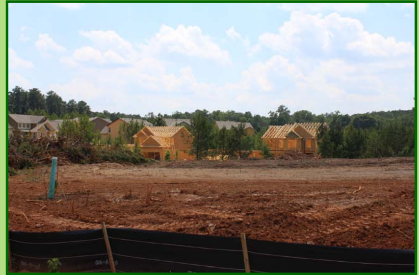
New single-family development off of Lester Road
