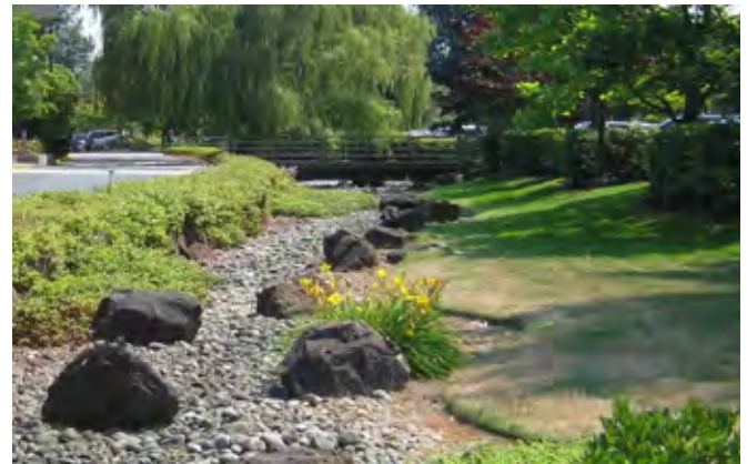
Encouraging bioswales and other ecological design solutions can help promote positive stormwater management
