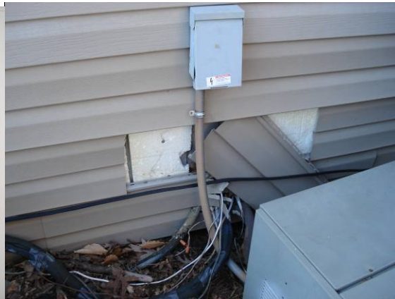
Faulty wiring
