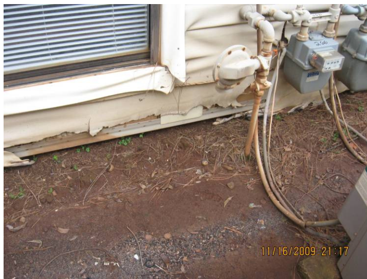
Damaged siding
