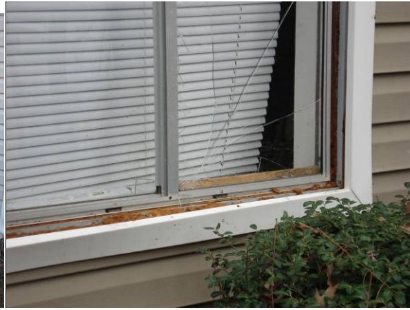
Broken window and rotting sill
