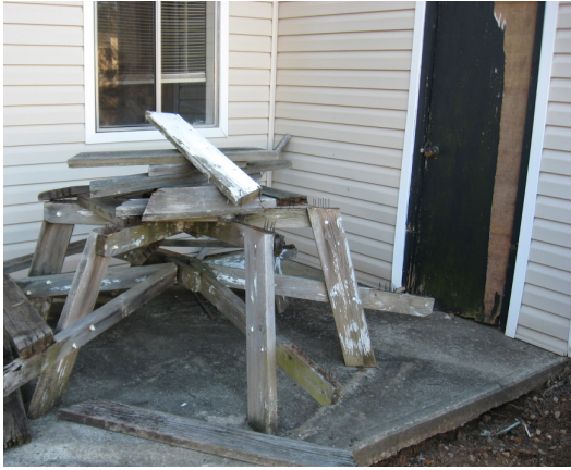
Debris, shearing under pad, rotten door
