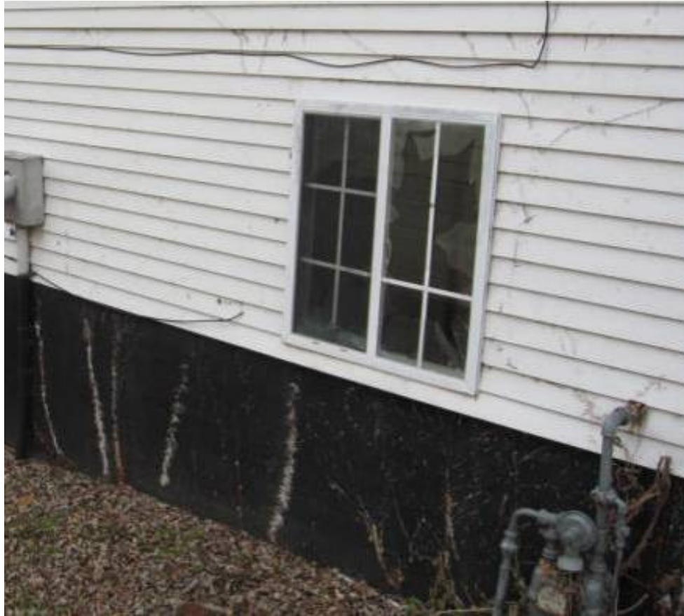
Broken basement window, vines removed
